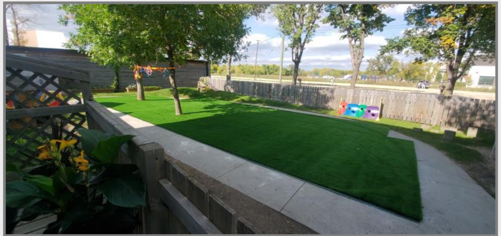
Daycare Play Yard Renovation, 2025
